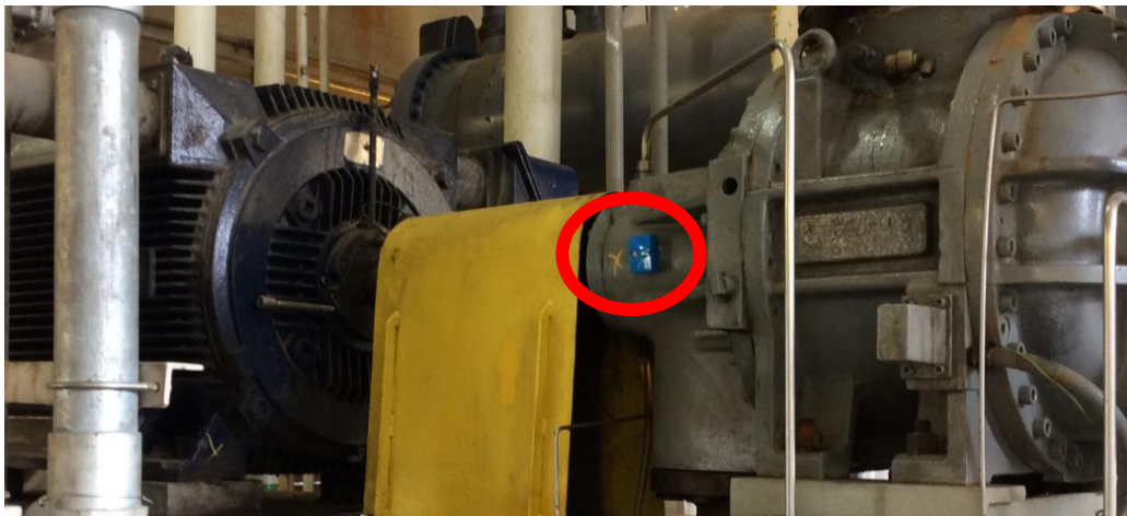
Figure 22: Vacuum Pump, side mounted to bearing housing
